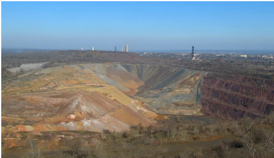
Figure 1 Rockfilling of the open pit #2 of PJS Central Mining and Enriching Combine with overburden rocks [13]
